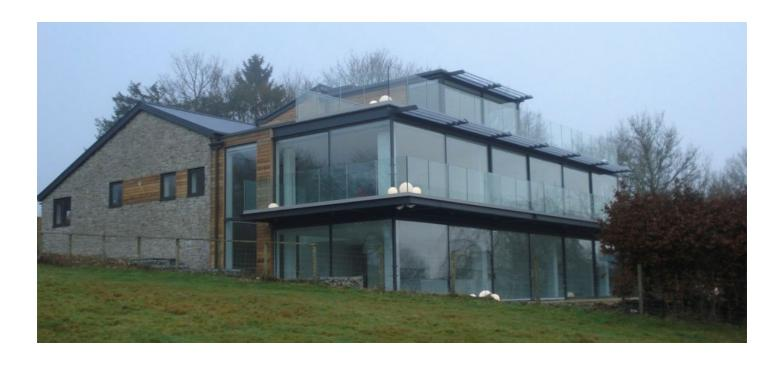
The front and side elevations were finished with a combination of ragstone walling and cedar cladding, whilst glazed curtain walling and sliding doors were specified for the rear elevation of the property. The glazing was continued into the balustrades to balcony / roof terrace areas.
